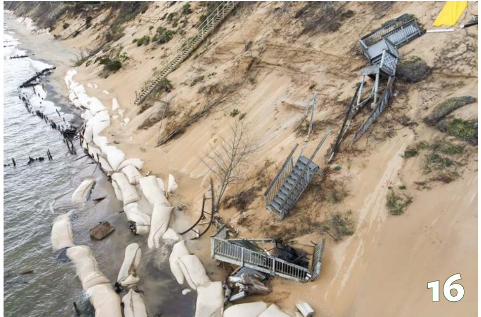
Aerial view of damage on eroding dune on Lake Michigan. Photo by Sarah Rypma.
