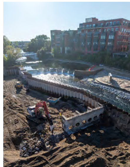
Construction of the fish-sorting channels underway at FishPass. Photo courtesy of Team Elmers.
