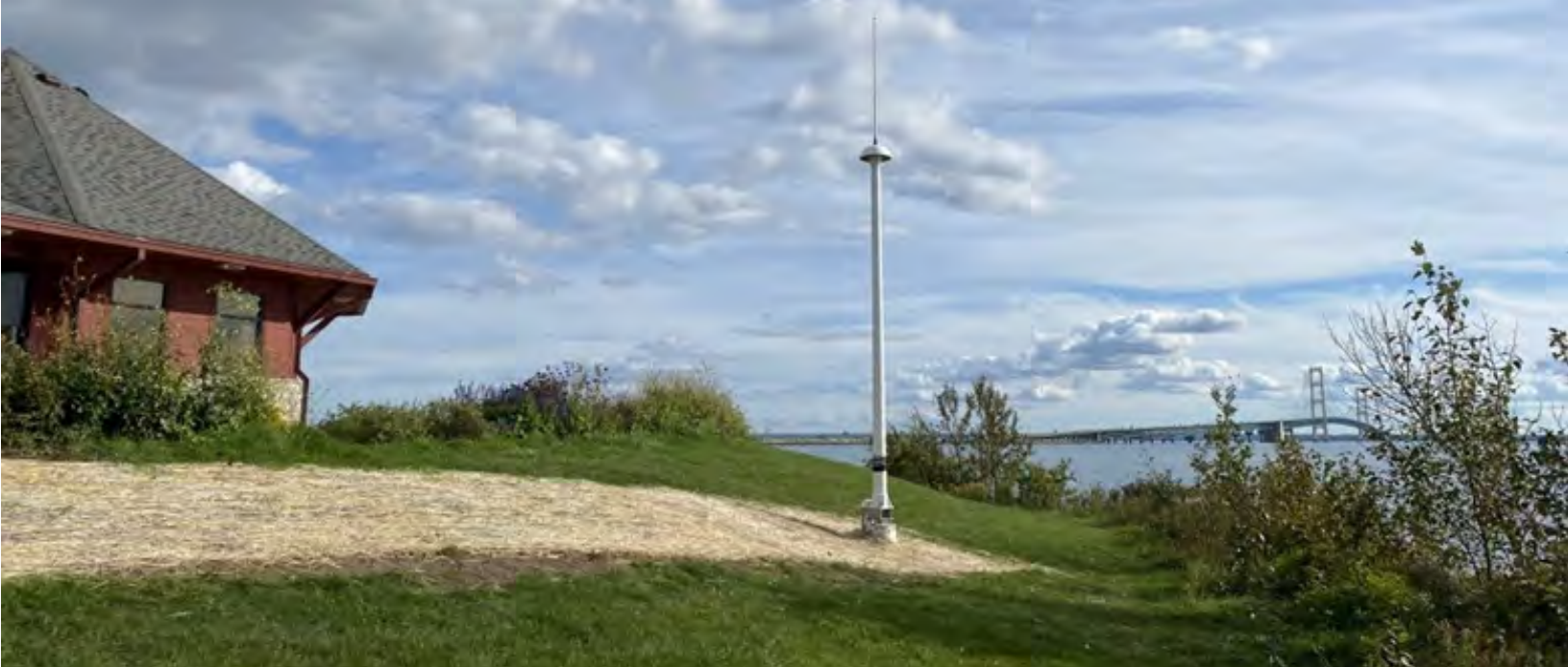
High-frequency radar antenna located at Bridgeview Park in St. Ignace, Michigan, overlooking the Straits of Mackinac.
