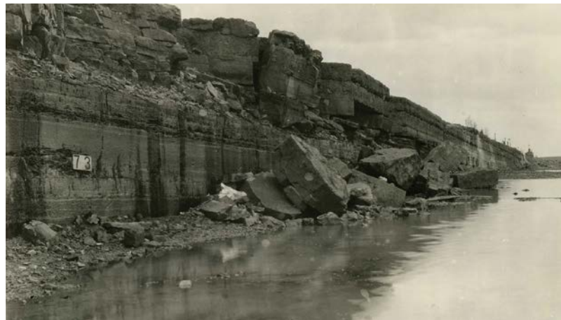
The Detroit River's dewatered Livingstone Channel features formidable bedrock and limestone formations in this 1933 photo. Between 1907 and 1912, a massive widening and deepening project took place in the 12-mile channel. Cofferdams were built to hold back the water, and dynamite was used to blast out bedrock and limestone. Additional deepening and widening projects occurred in the 1920s and '30s. Photo credit: U.S. Army Corps of Engineers.
