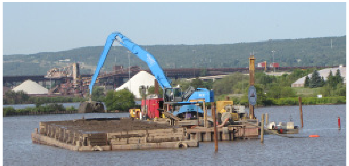
Contaminated sediment remediation in the St. Louis River, Duluth, Minnesota. Credit: Minnesota Pollution Control Agency.
