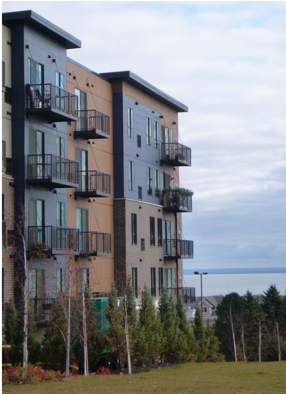
ENDI mixed-use development overlooking Lake Superior and steps from the Duluth Lakewalk. Credit: U.S. Environmental Protection Agency.
